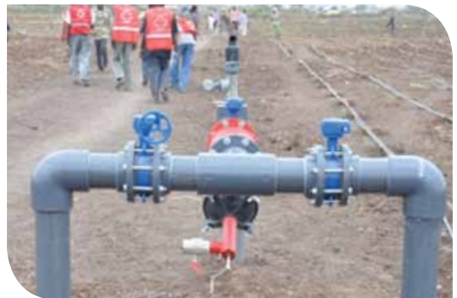
The water and irrigation infrastructure in Waldaa, Moyale on the Kenyans for Kenya farmland
